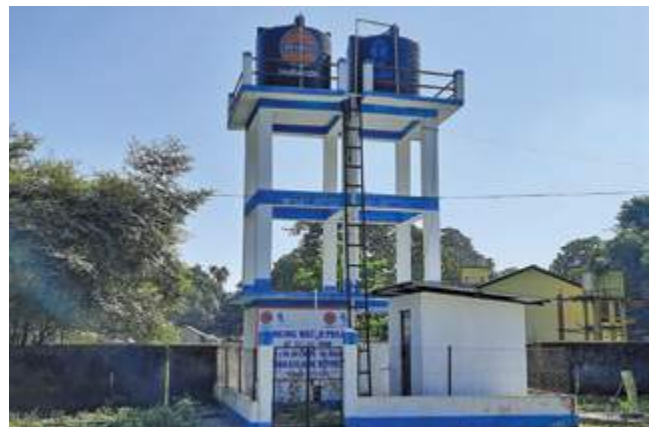
Drinking Water Project, Bishnupur, Bongaigaon in Assam
