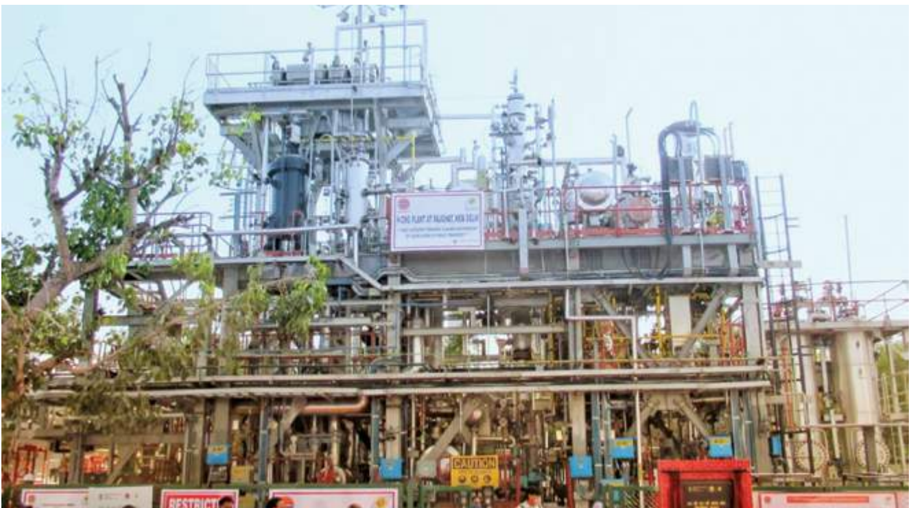
Hydrogen CNG plant at Rajghat, New Delhi
