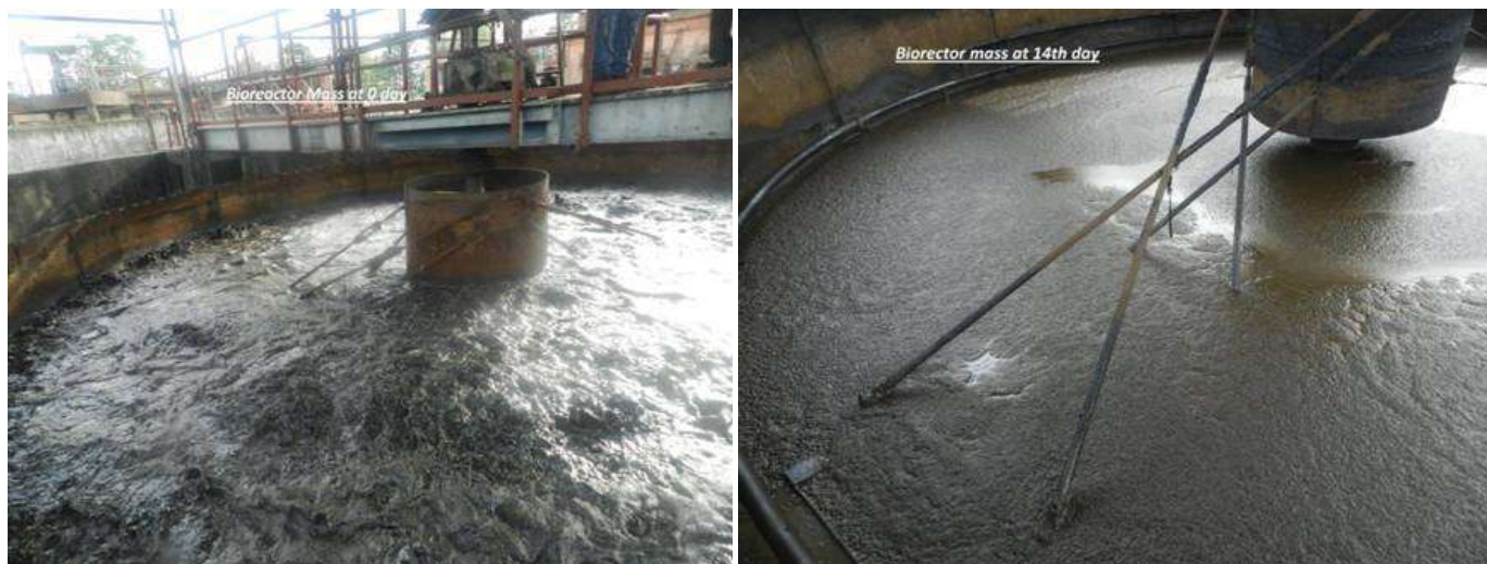
Bio-remediation facility of BGR
