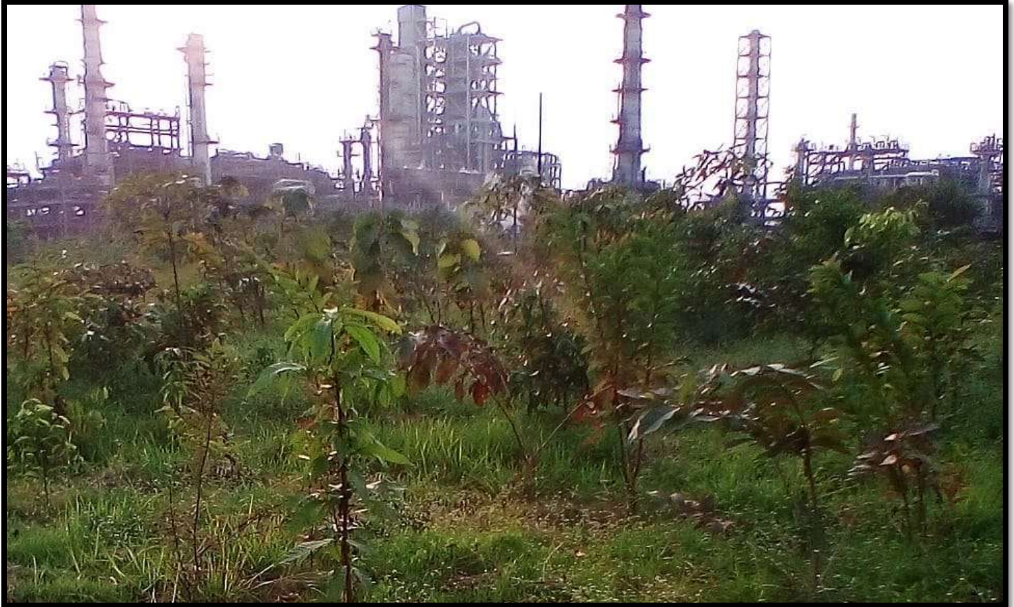
Planted on Aug,2021, in the complex, North side of new project(IndMax & BS-VI), Growth as on Mar,2023
