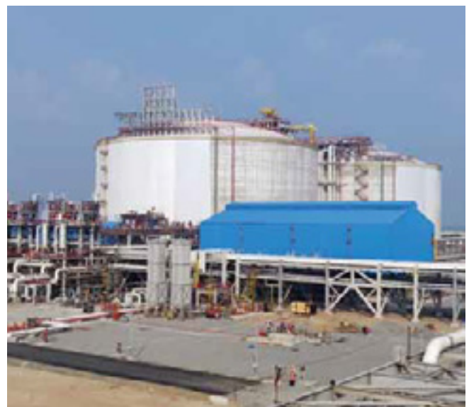
IndianOil's 5-MMTPA terminal at Ennore for LNG imports and sourcing more LNG directly to meet the increasing domestic requirements.
