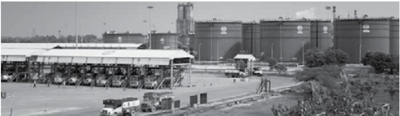
Leveraging technology, IndianOil introduced a pioneering concept of Smart Terminals with a centralised automated system at its supply points, that takes care of all core operations, thus enabling manpower to focus on critical maintenance and safety-related support.
