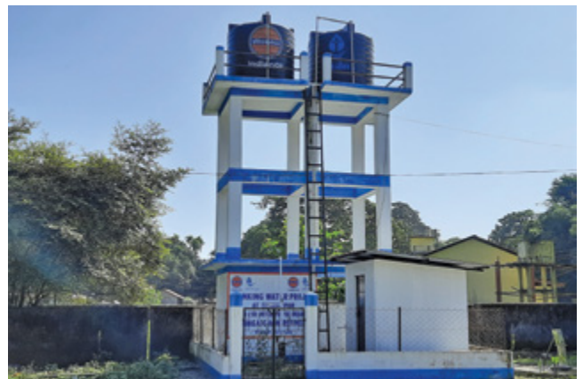
Drinking Water Project, Bishnupur, Bongaigaon in Assam
