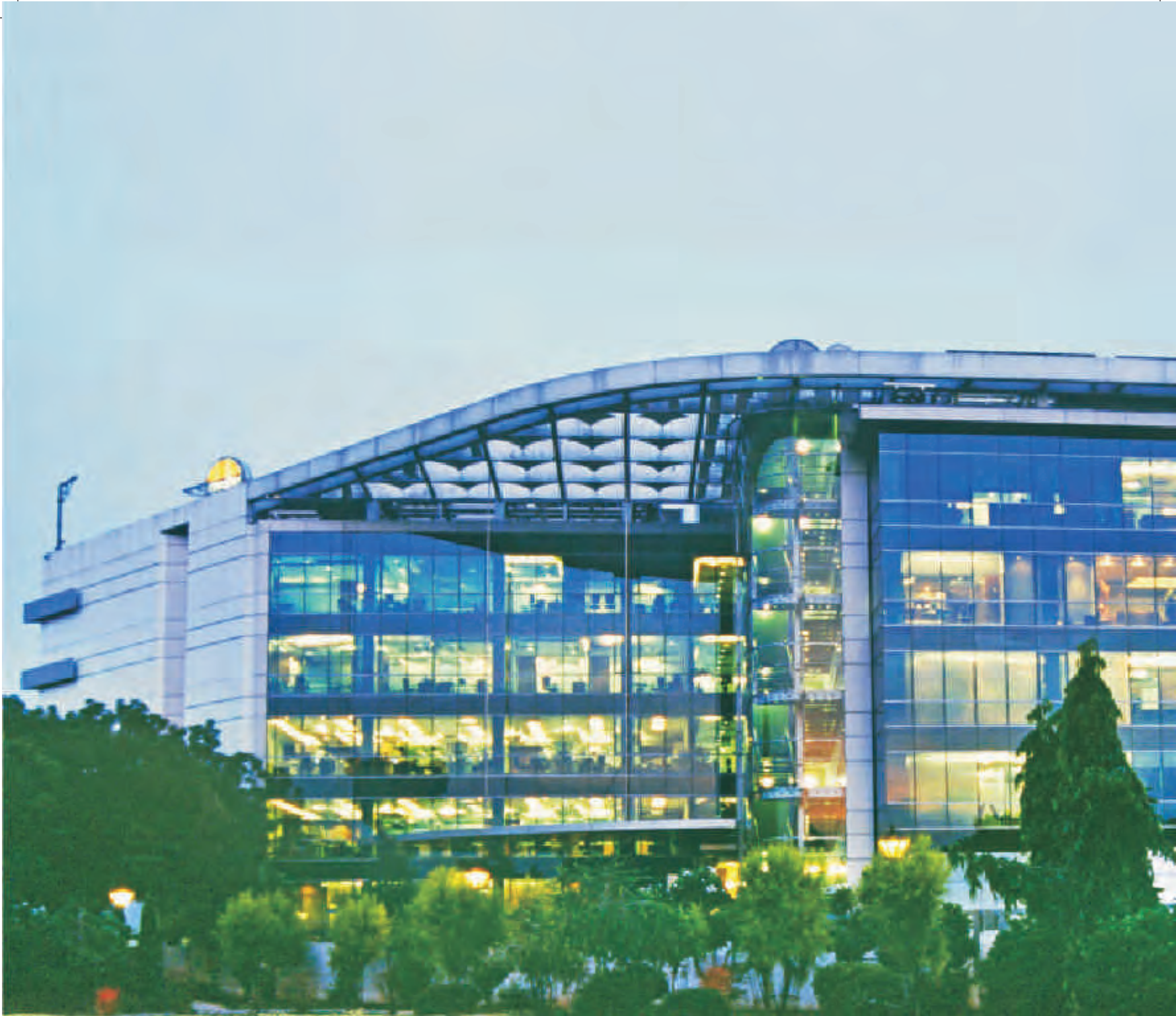
New age design - IndianOil's energy efficient and eco-friendly office at New Delhi
