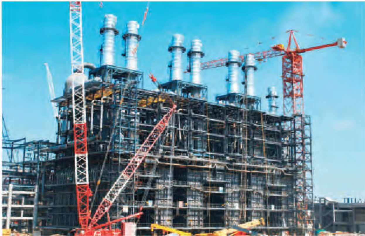
Construction of Naphtha Cracker Unit at Panipat Complex
