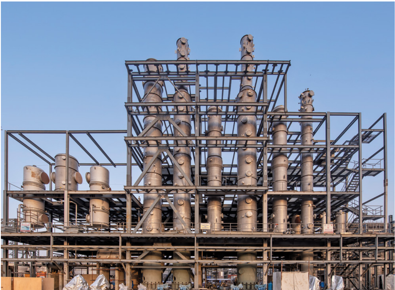
Upcoming 2G Ethanol plant at Panipat
