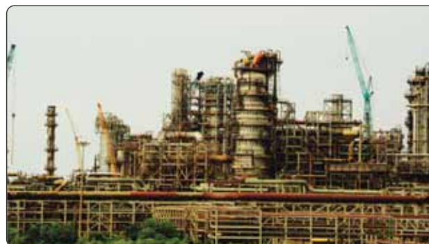
IndianOil's Paradip Refinery in Odisha under commissioning.
