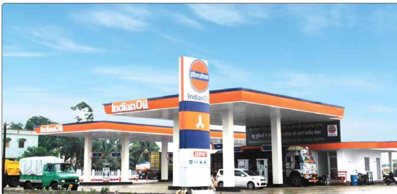
IndianOil's new large-format fuel station at Haldia.
