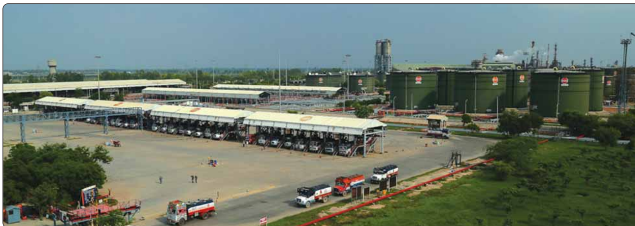
IndianOil's products bulk storage terminal at Panipat.
