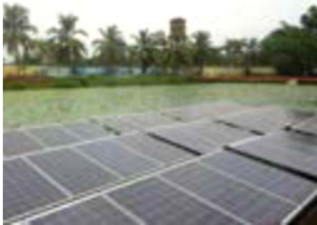
IndianOil's floating solar plant at Cochin Bottling Plant. The floating structure is made of 80% recycled metal.
