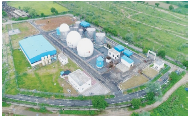
100 TPD Compressed Biogas Plant at Hingonia, Jaipur
