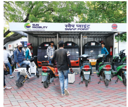
A battery swapping facility by IndianOil and Sun Mobility
