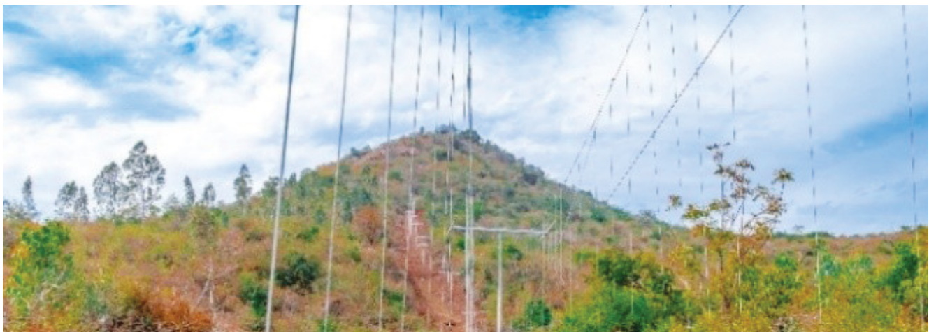
Solar Tentacle Fencing installed at Kaundinya Wildlife Sanctuary, Chittoor, AP
