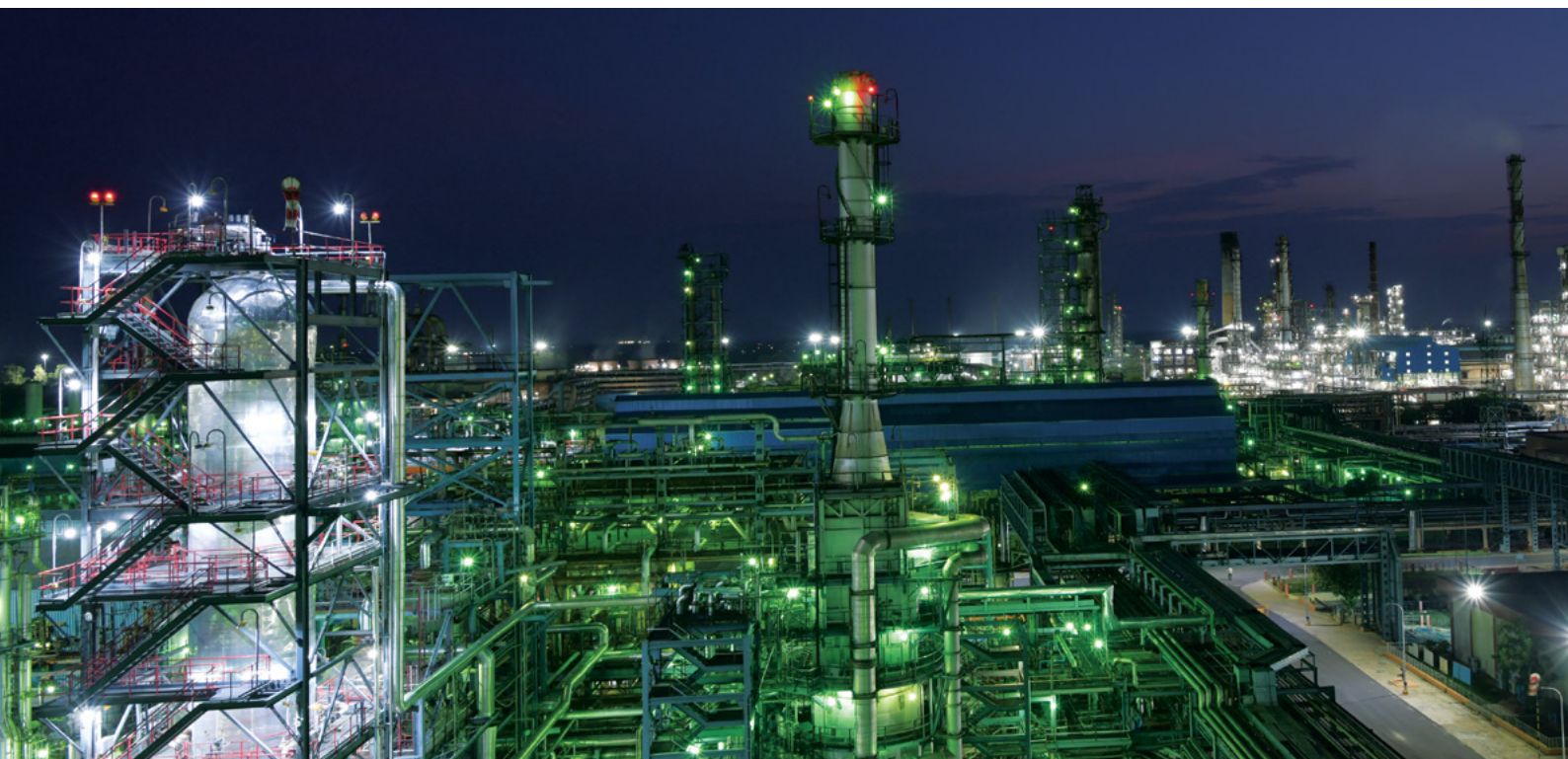
Night view of Mathura Refinery
