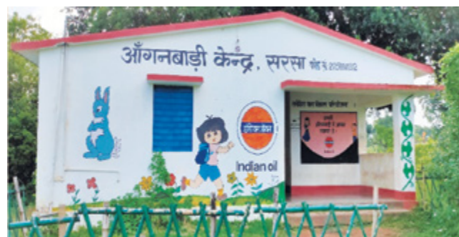
Renovated and upgraded Anganwadi Centre in village Sarsa, Deogarh, Jharkhand
