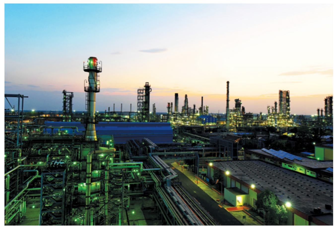
A view of IndianOil Mathura Refinery
