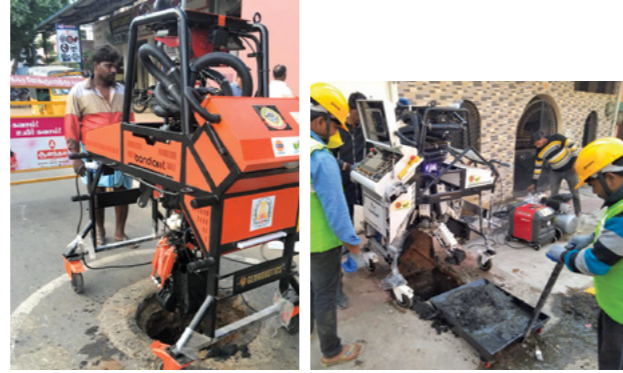
Bandicoot robotic machine handed over to eliminate manual scavenging of sewers
