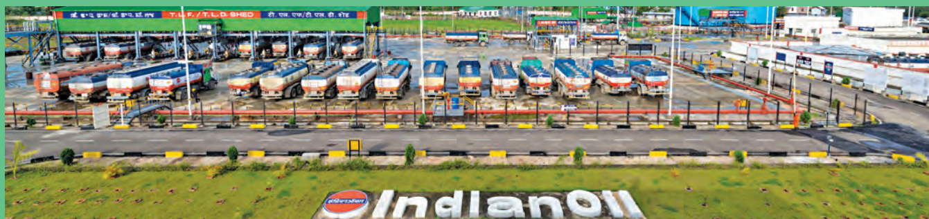
IndianOil's bulk storage depot at Chingmeirong, Imphal with a storage capacity of 6,700 kl.
