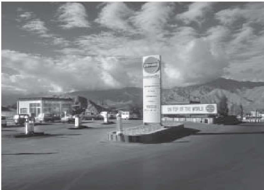
Ladakh Filling Station at Leh, as it looks now - IndianOil serves the people even in the remotest corner of the country.
