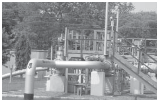
An installation of Panipat-Bhatinda pipeline.
