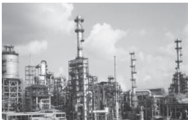
PX-PTA plant of Panipat Refinery.
