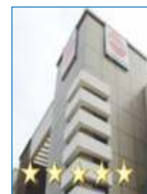
Indore Divisional Office Building
