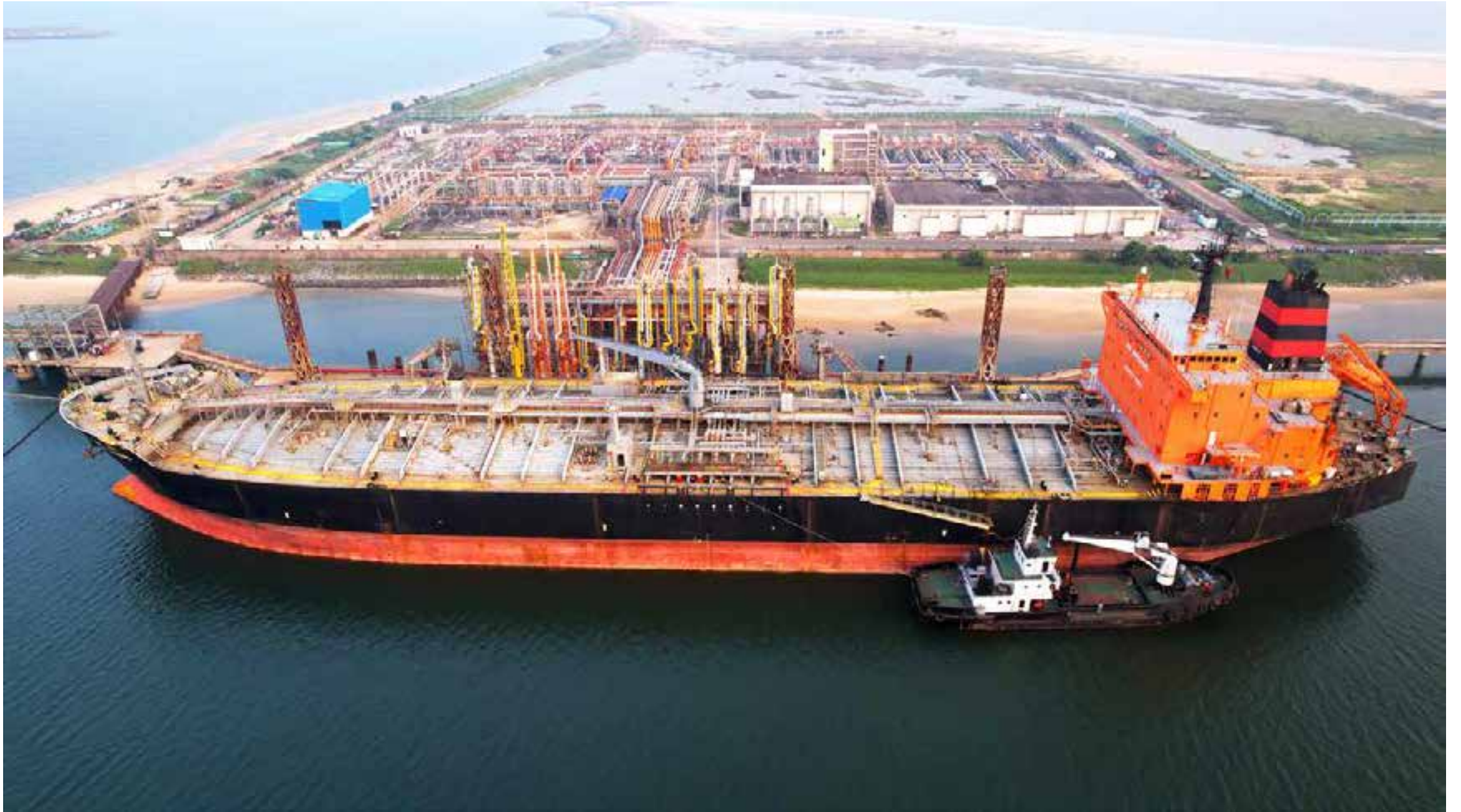
North Oil Jetty at Paradip
