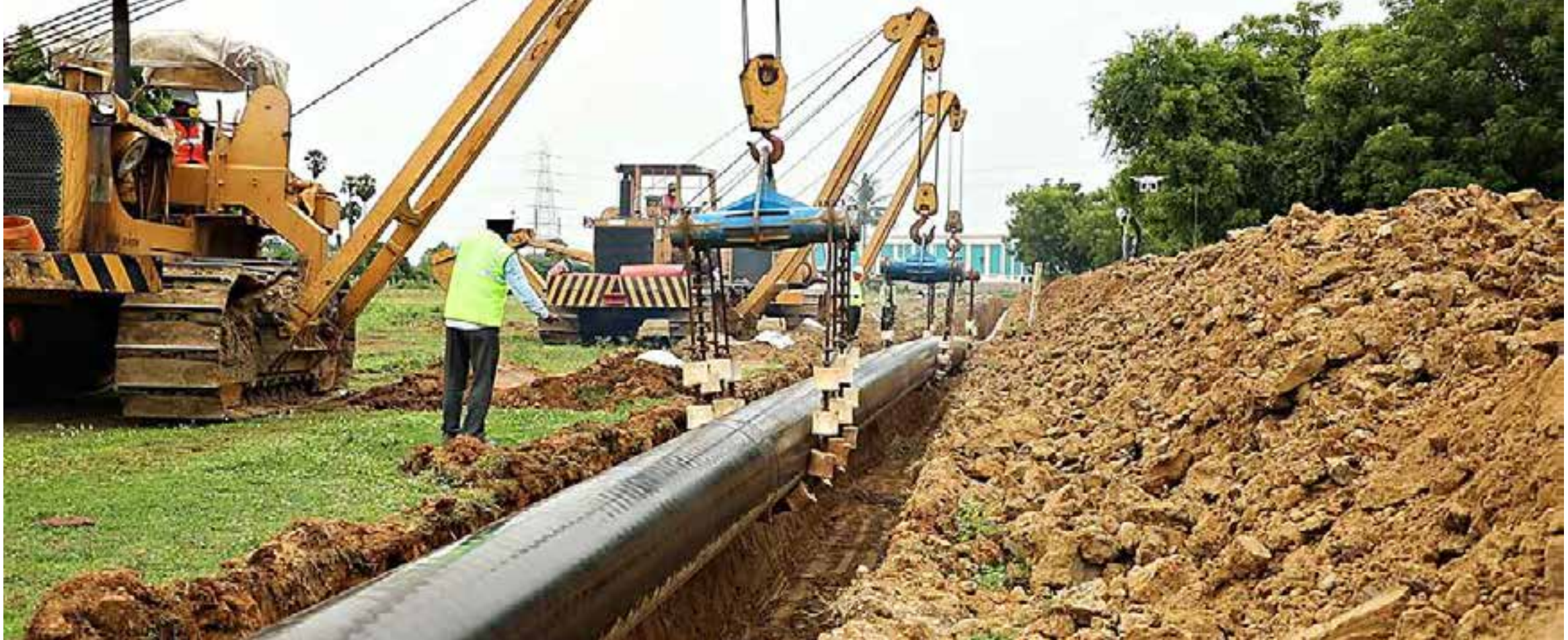
Lowering of pipeline in progress
