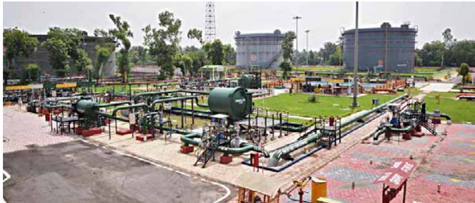
ATF Seperator Filter at NRPL, Bijwasan
