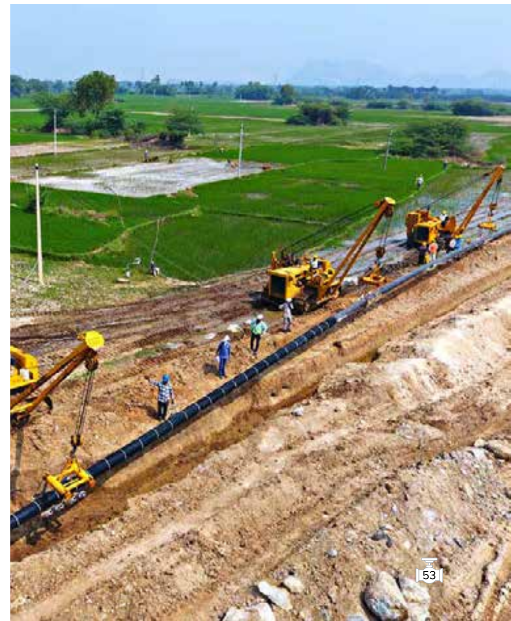
Mainline Lowering in Progress, Vijayawada
