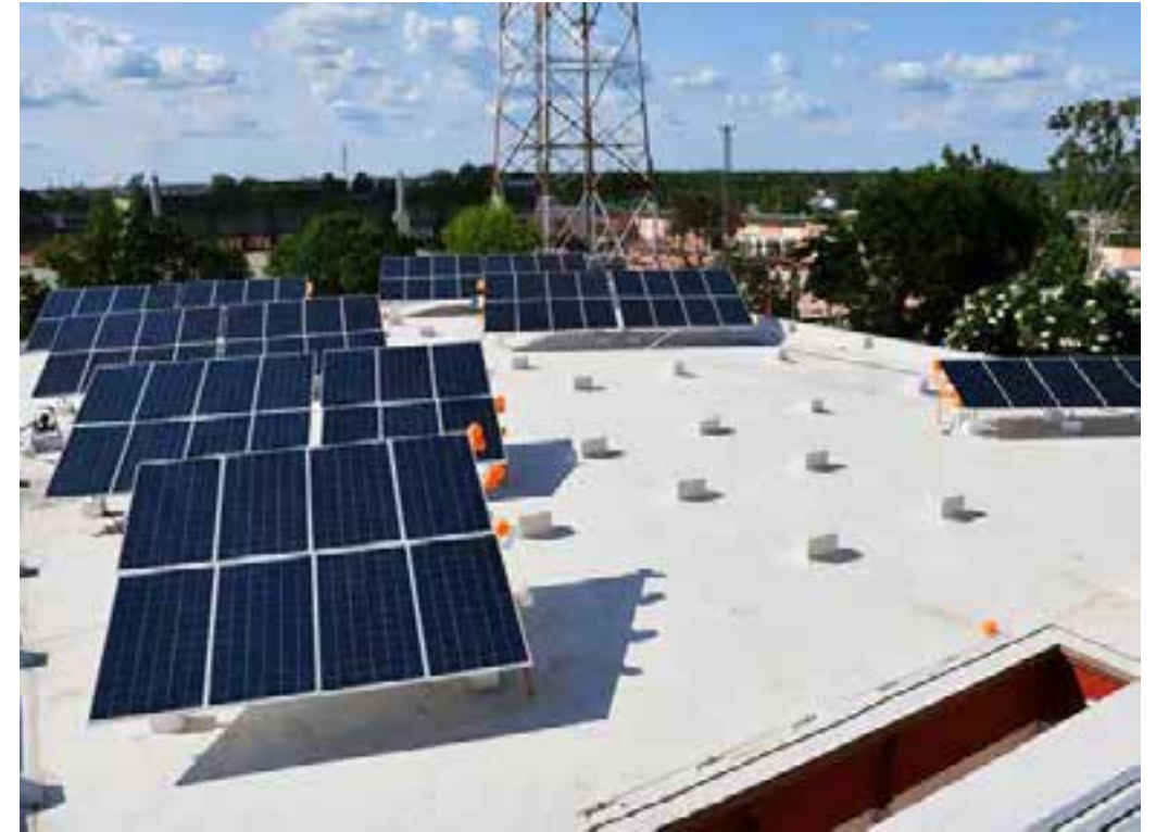
30 KW SPV Plant at WRPL Gauridad
