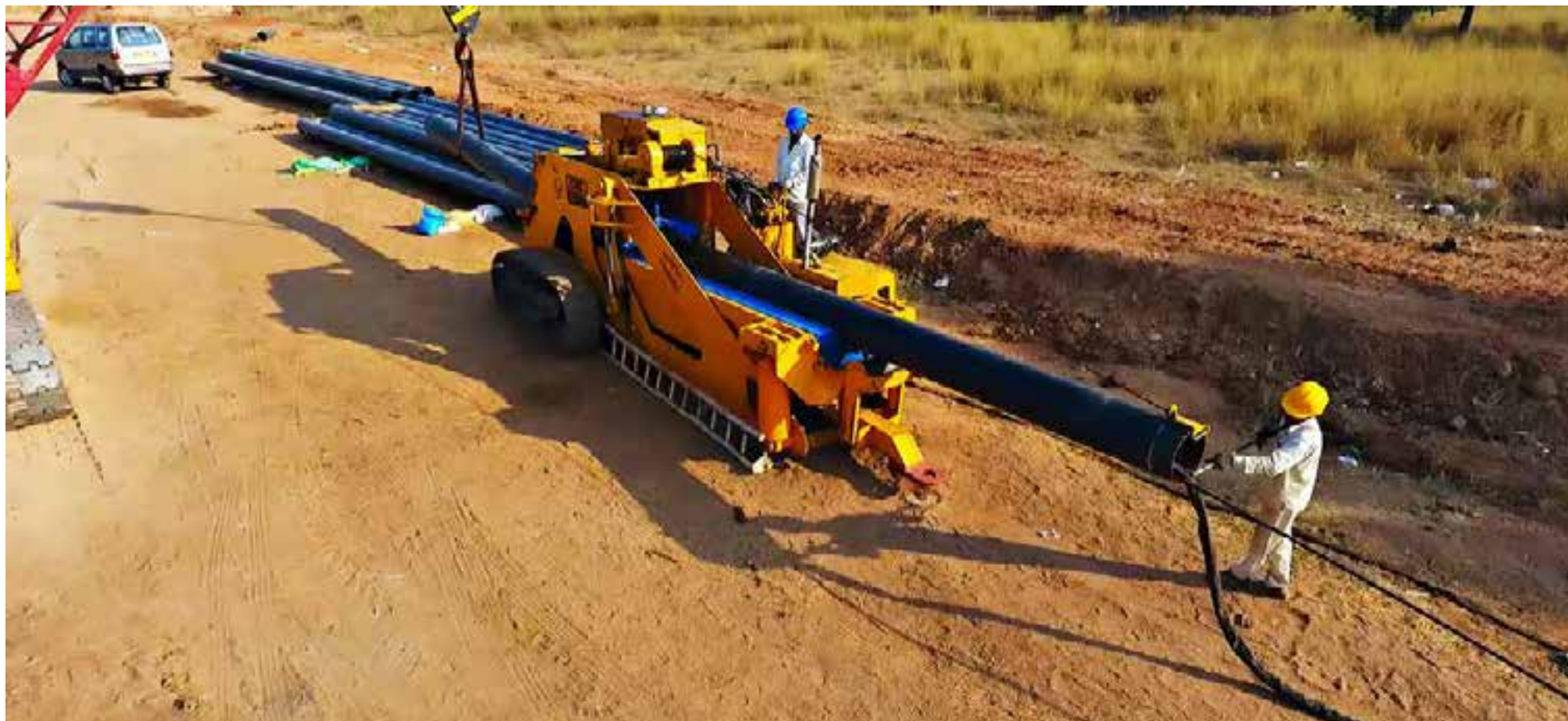
Pipe bending in progress
