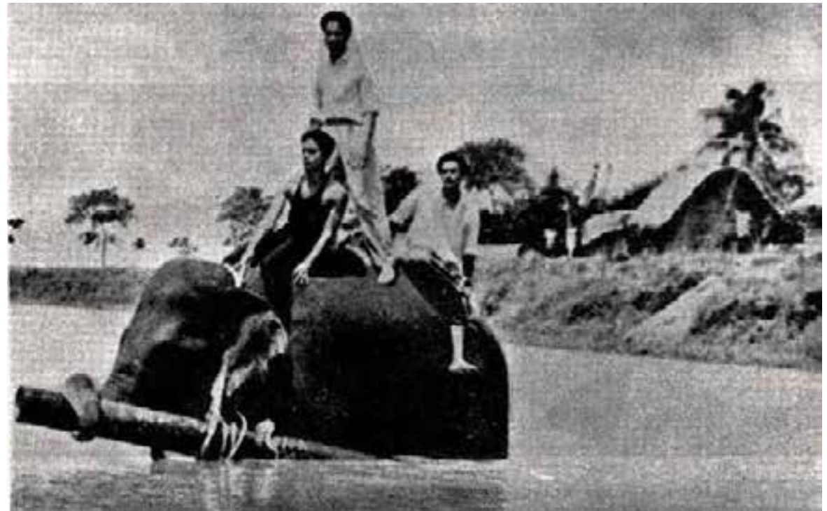
Laying of pipelines for transporting refined petroleum products involves cumbersome operations. Trained elephants were utilised in Assam to ferry pipelines across the rivers
