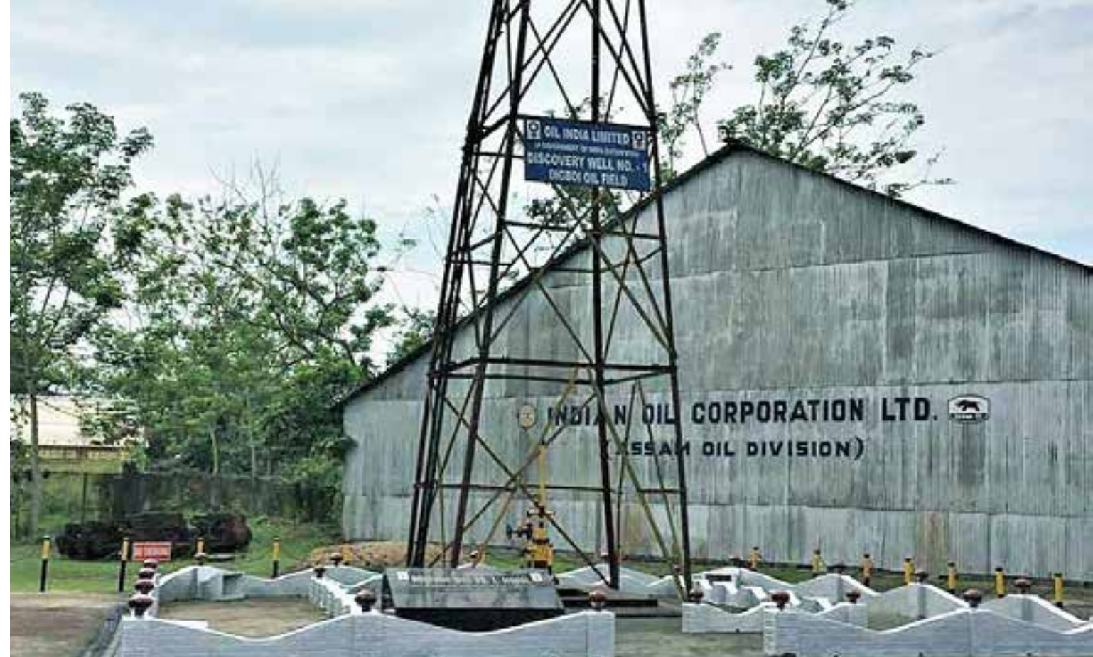
Digboi's first commercial oil well, now preserved as a monument, began production in November 1890
