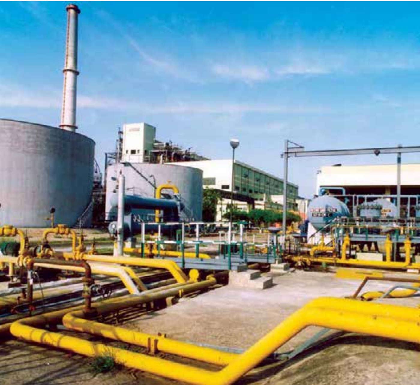
Pipeline Infrastructure including Pump Shed, Tank Farms, Piping
