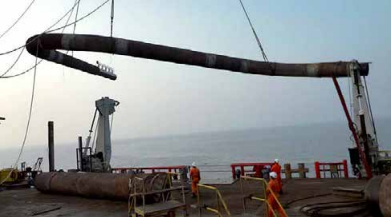
Lifting in progress of Extended Portion of Pipeline for Route at Paradip
