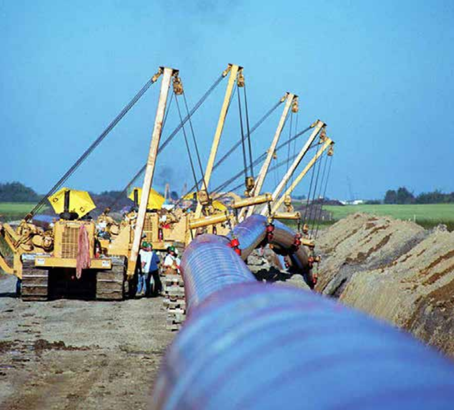
Mainline Lowering in Progress, Vijayawada
