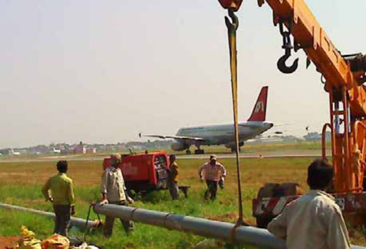
ATF Pipeline laying inside Chennai Airport
