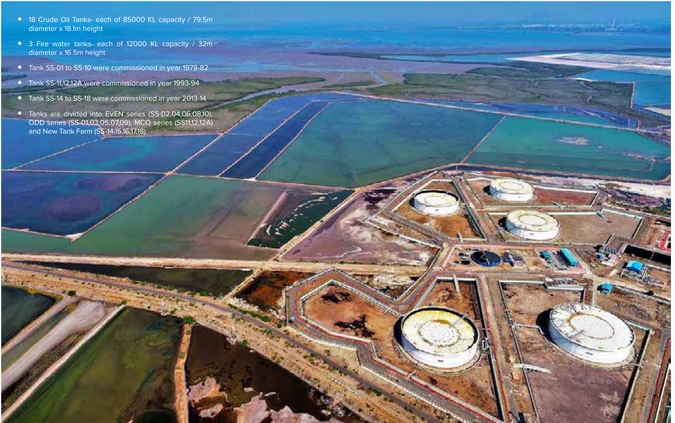
A view of Vadinar Crude Oil Terminal (storage tanks)
