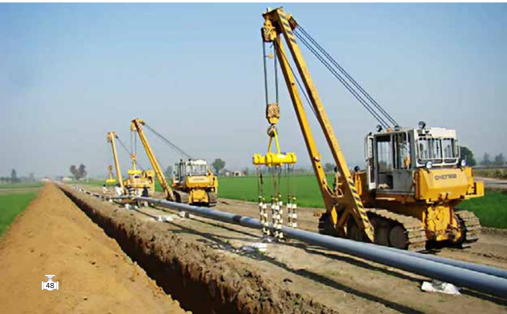
Lowering of Pipelines
