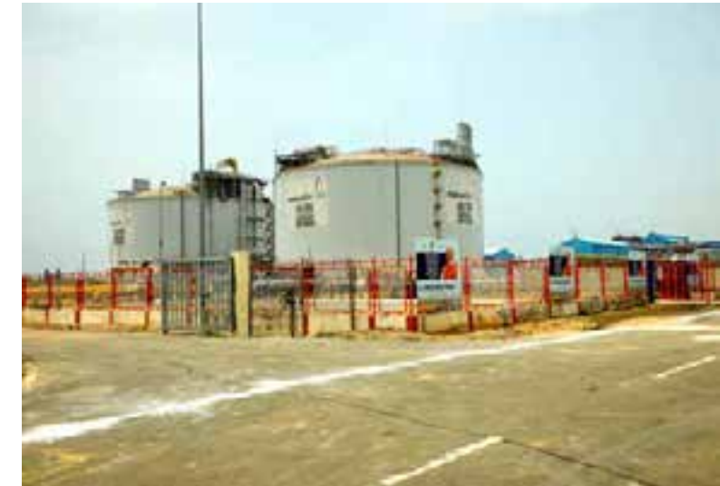
ETBPNMTPL - Longest Gas Pipeline
