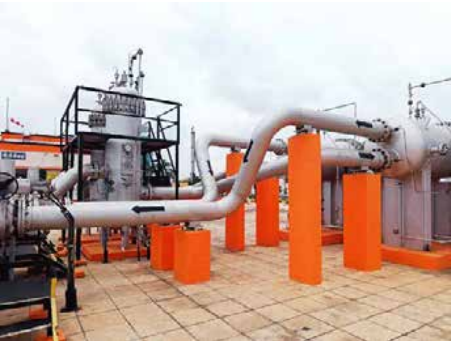
ATF Seperator Filter at PRRPL, Raipur
