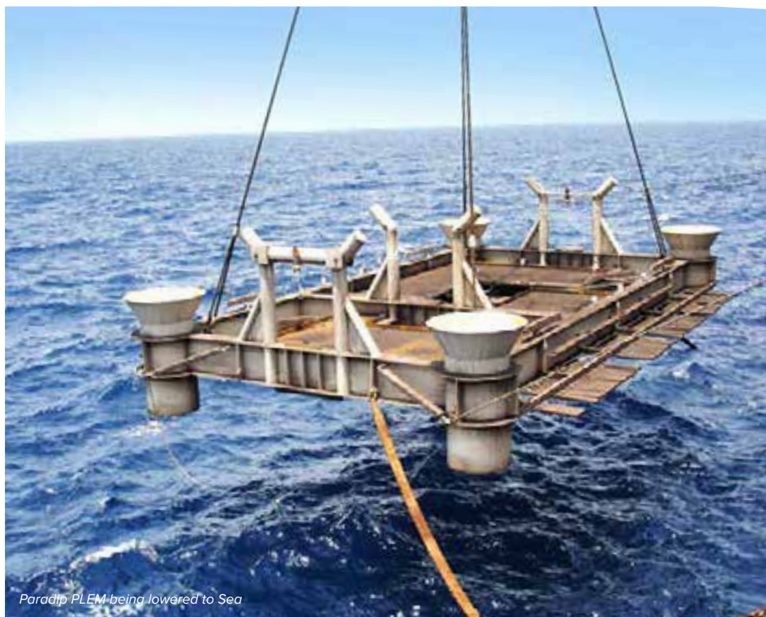
Lifting in progress of Extended Portion of Pipeline for Route at Paradip
