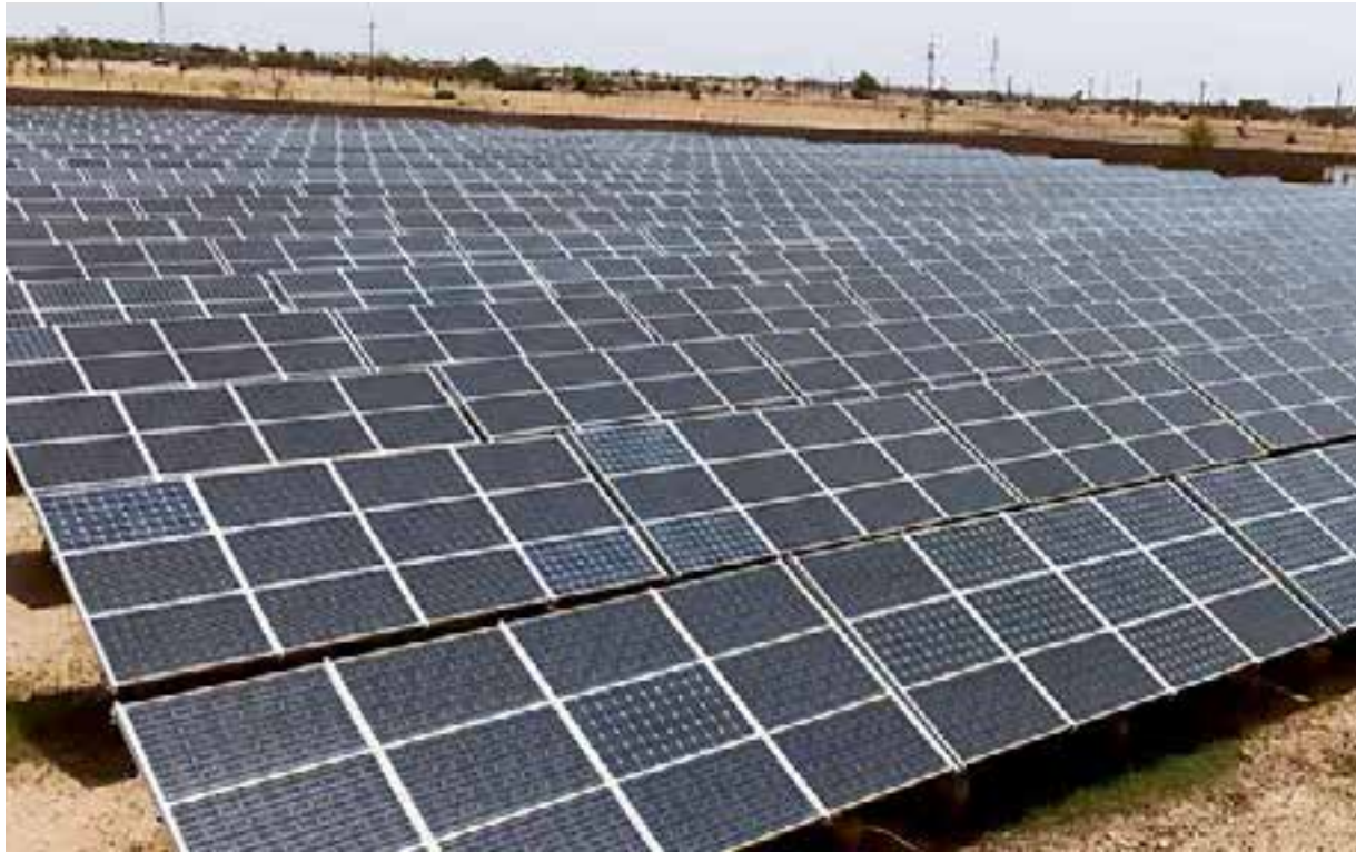
WRPL Rawara Plant: 5MW SPV Plant, Rawra, Rajasthan Commissioned in Jan-2012
