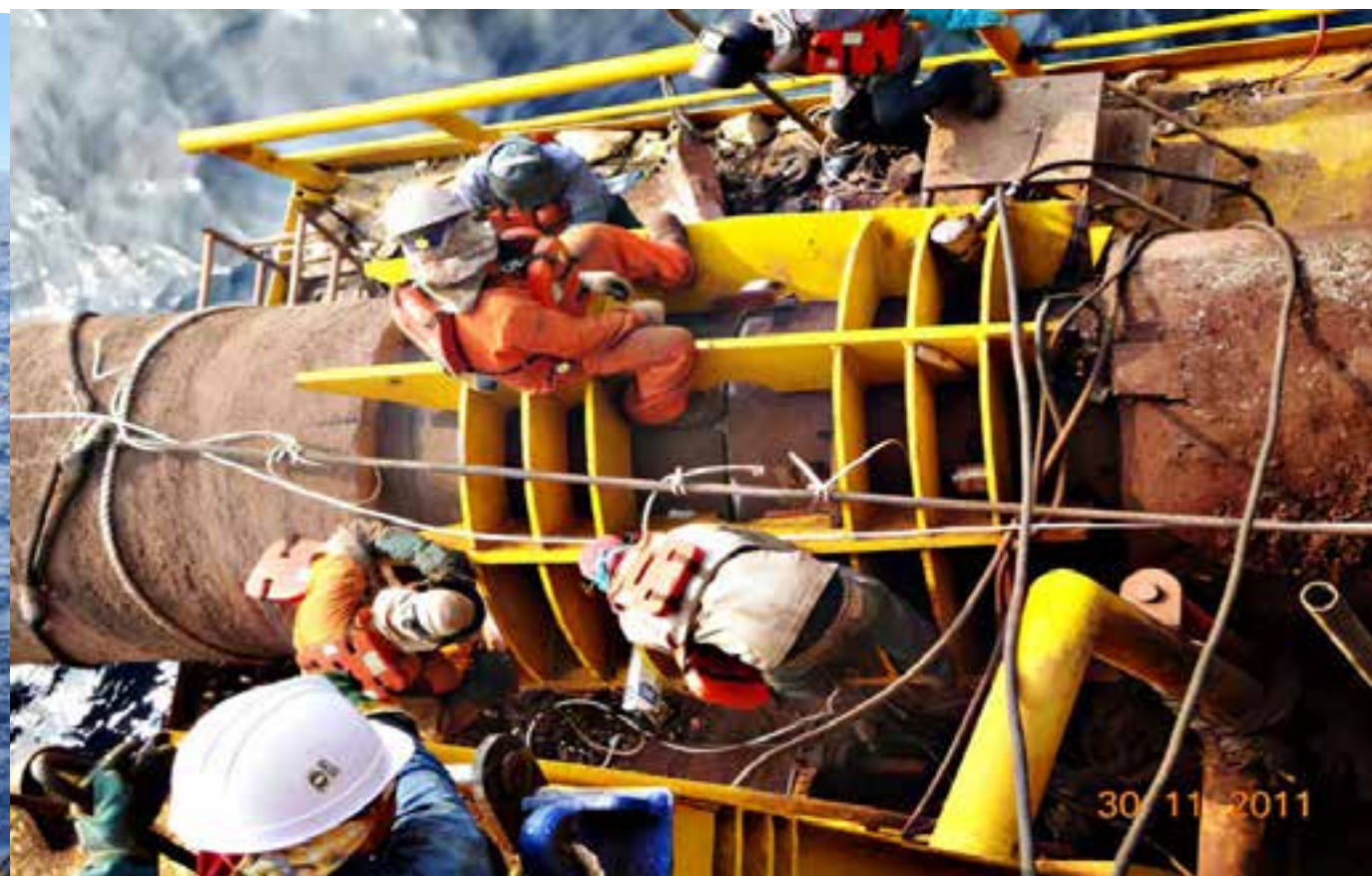
Welding is in progress at Paradip
