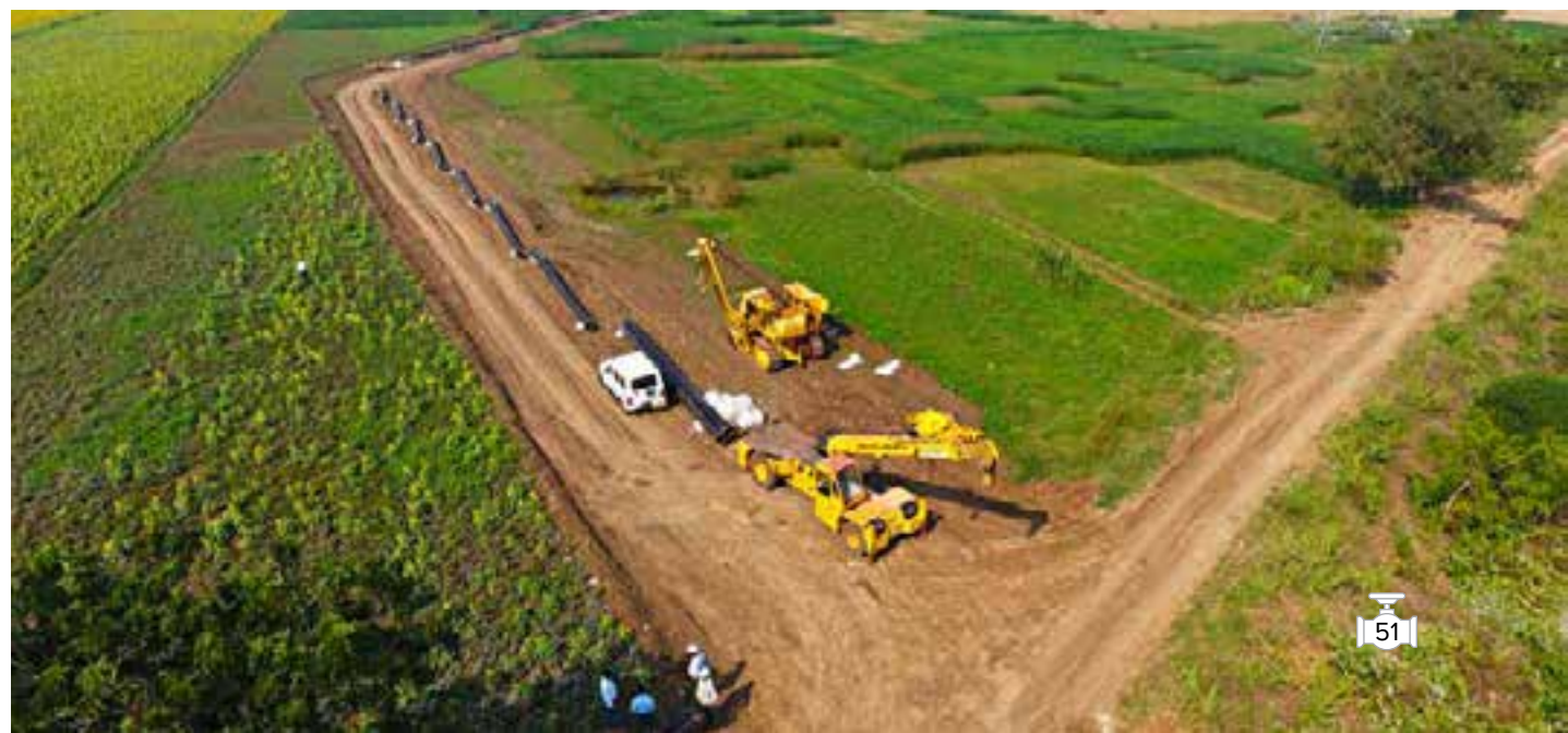
Stringing in progress, Vijayawada
