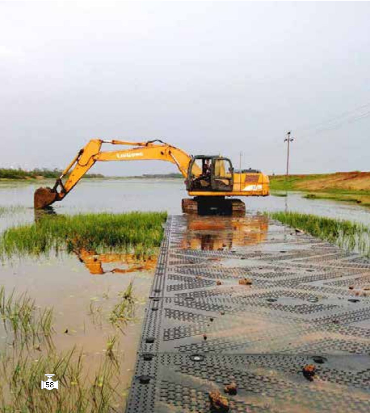
Use of Portadeck Mat in water logged area
