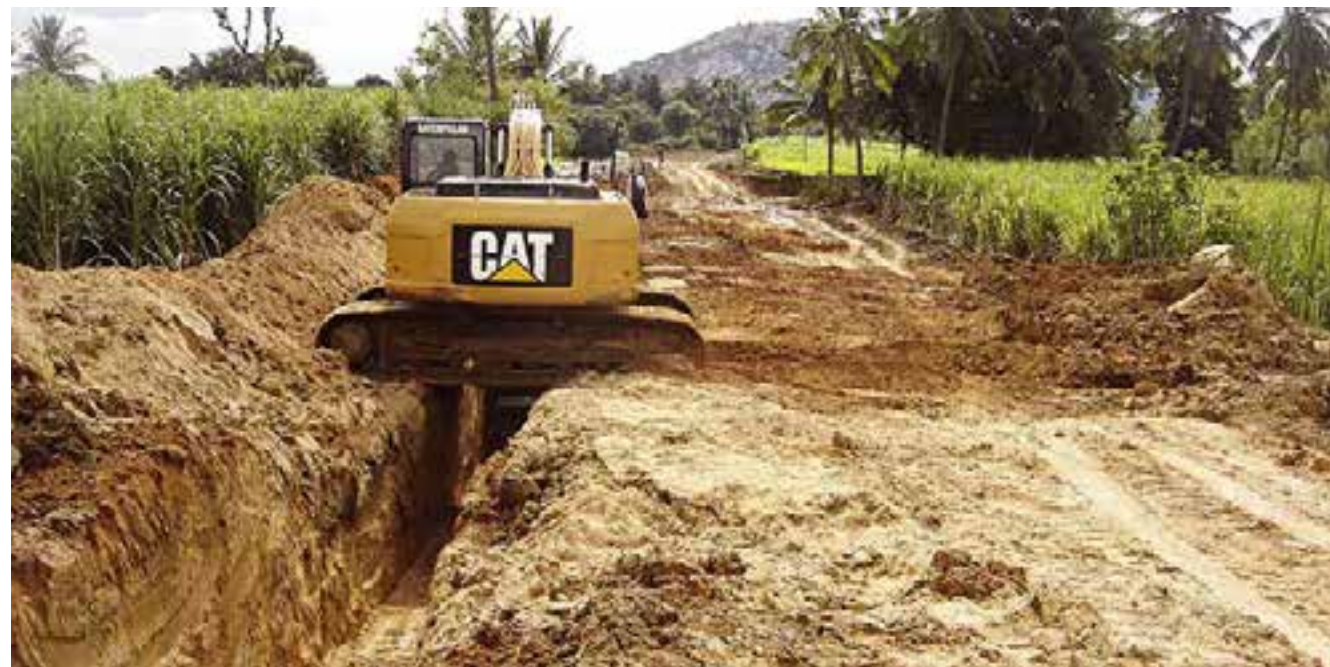
Trenching in progress
