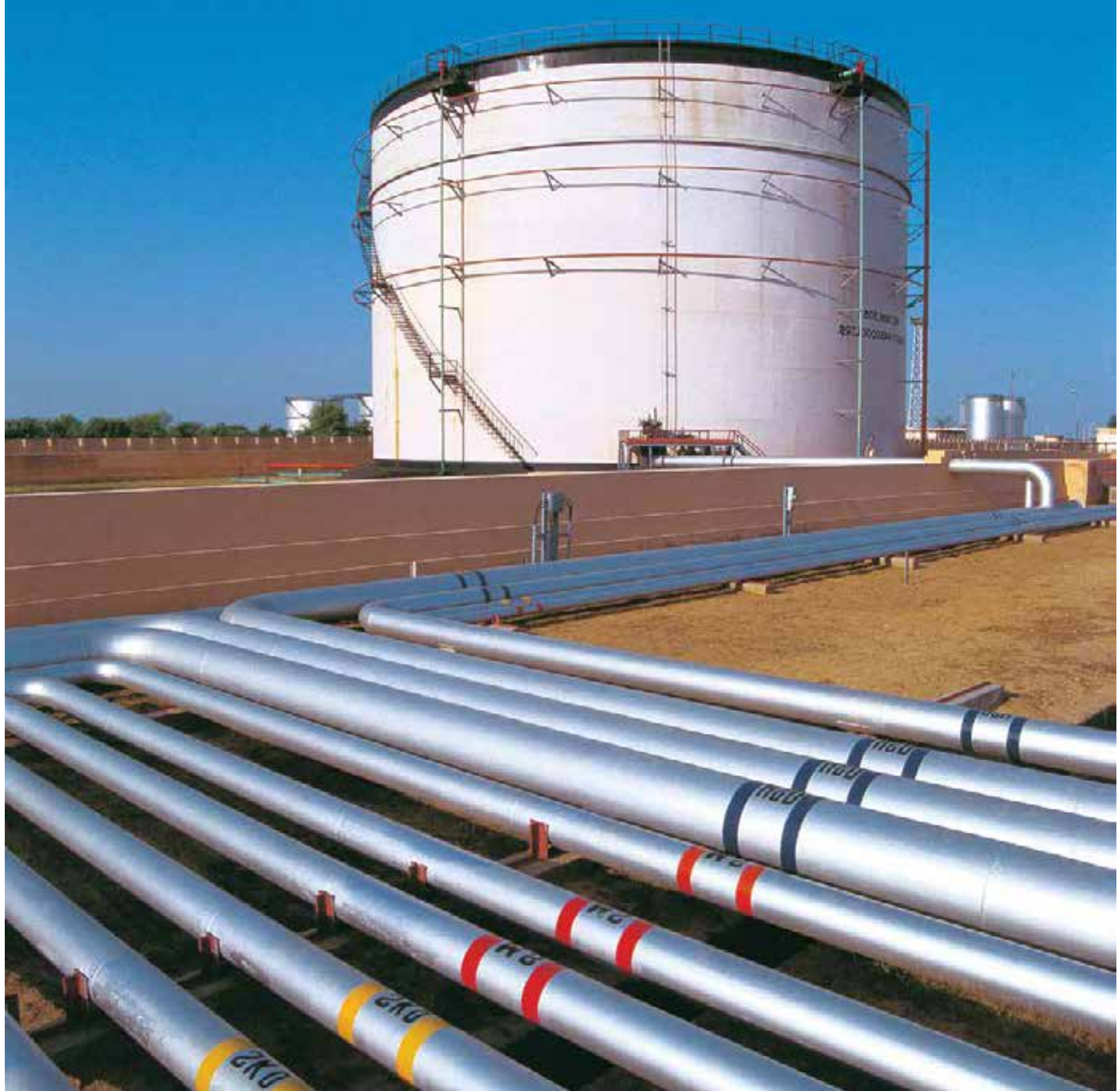
Product Transfer Pipelines
