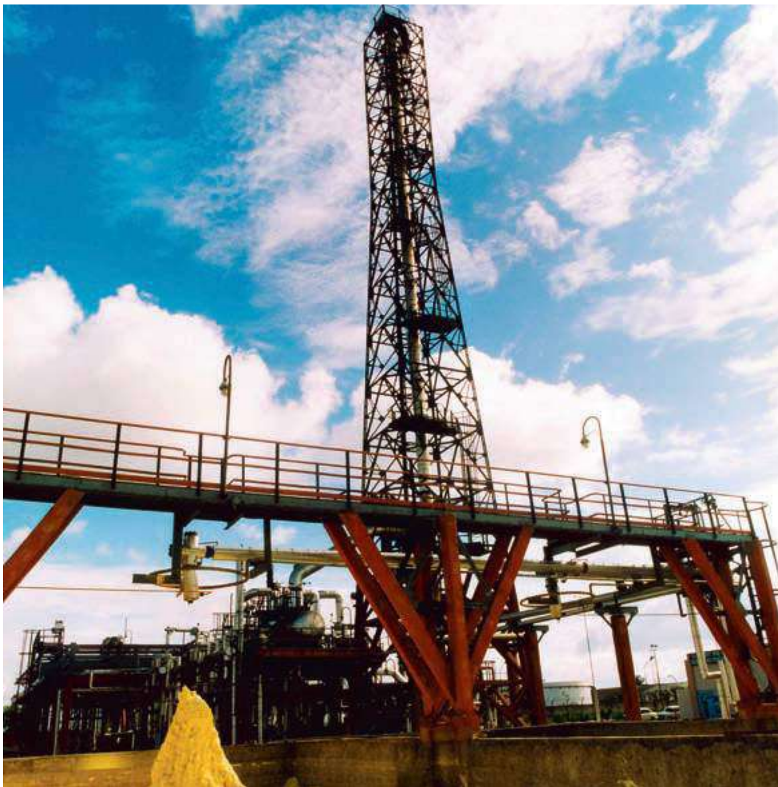
The high-efficiency sulphur recovery unit commissioned at Haldia (1994) enabled recovery of 96 per cent sulphur from flue gas.
