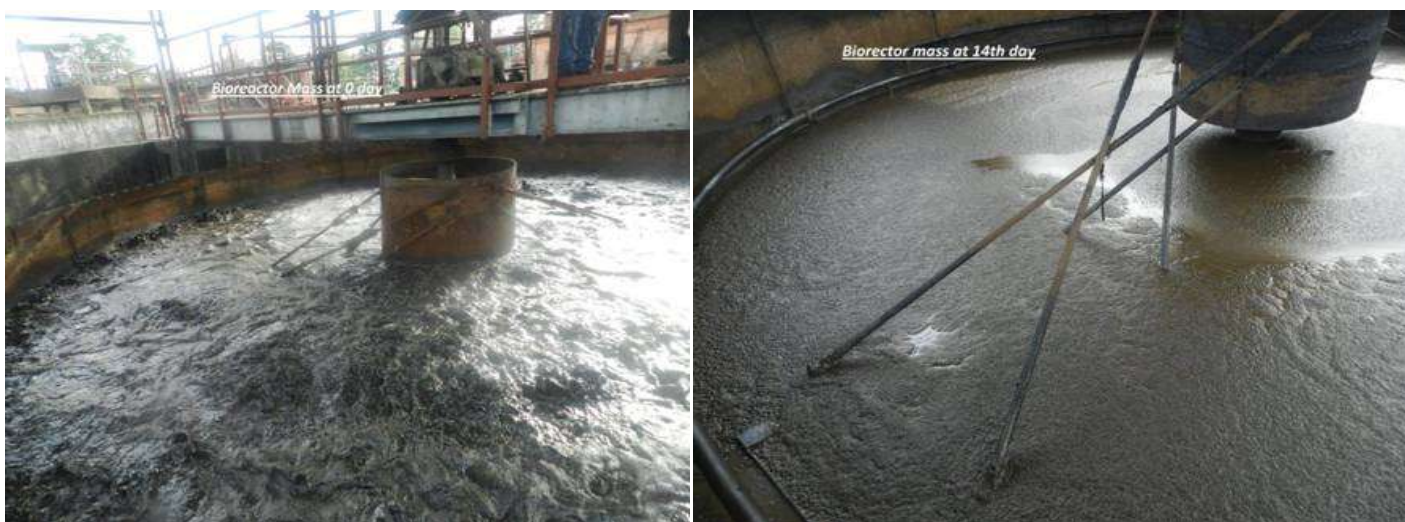
Bio-remediation facility of BGR
