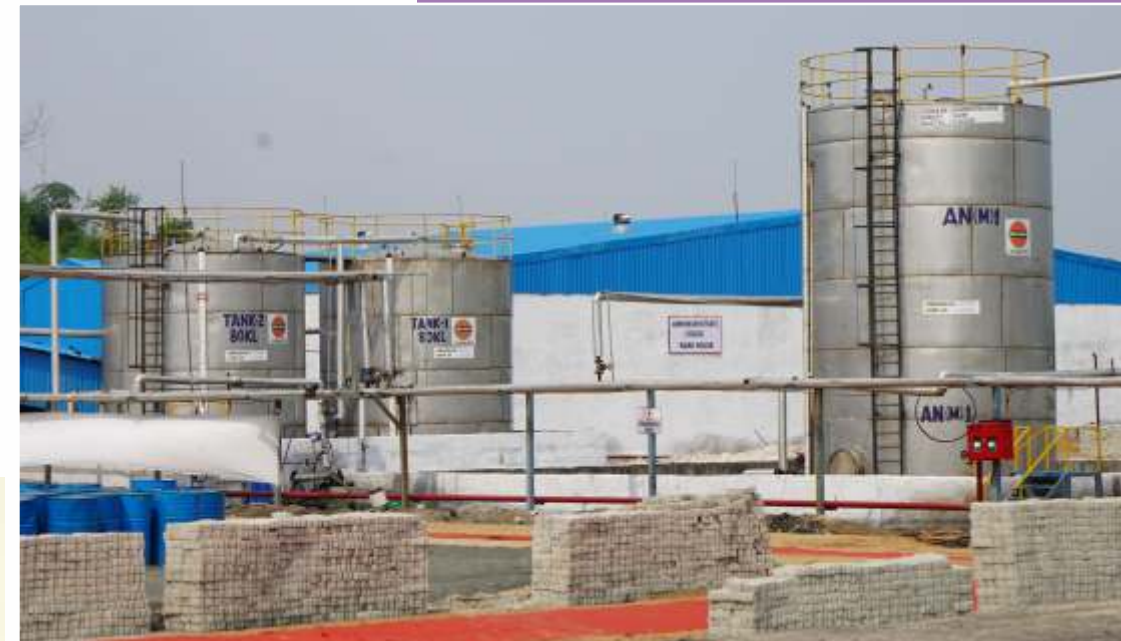
Ammonium Nitrate Melt Tank - Umrer
