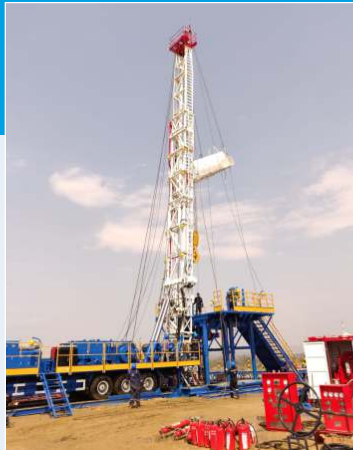
Completion Rig in operation in North Karanpura CBM block, India
