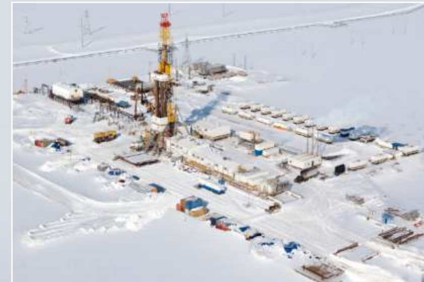
Drilling Rig in operation at Vankor field, Russia IndianOil has acquired non operating participating interest in this giant producing field in the year 2016. Current gross production of the field is around 254,000 boepd
