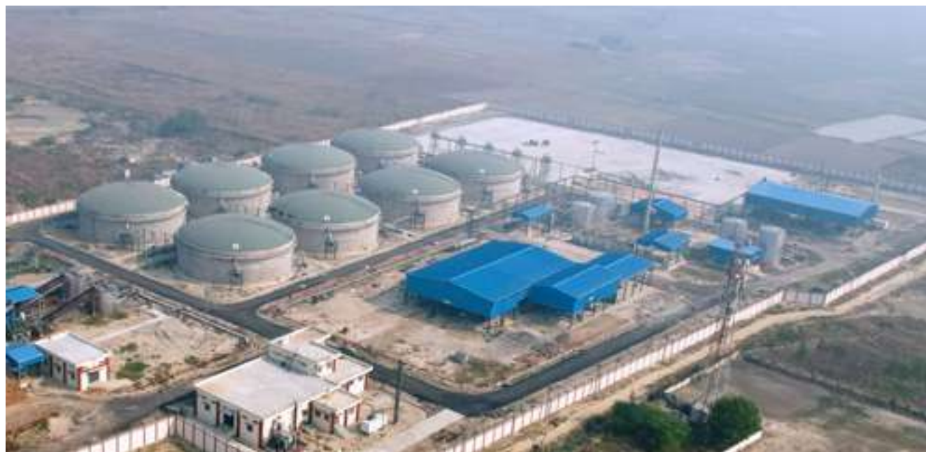
Aerial View of CBG Plant at Gorakhpur
