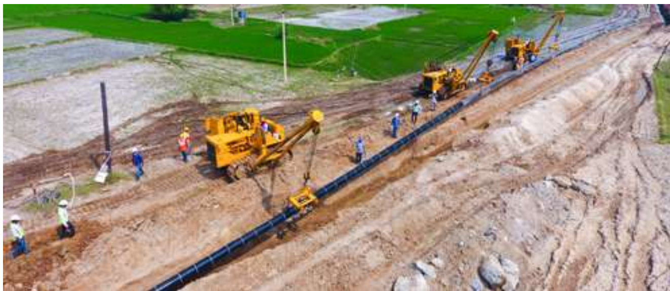
Mainline Lowering in Progress at Vijayawada, as part of Paradip Hyderabad Pipelines Project
