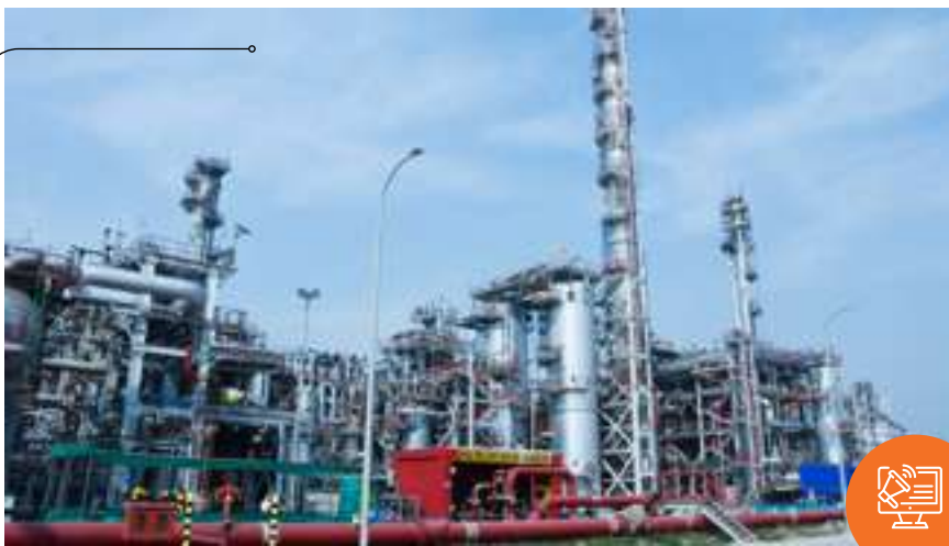
Ethylene Recovery Unit at Paradip Refinery
