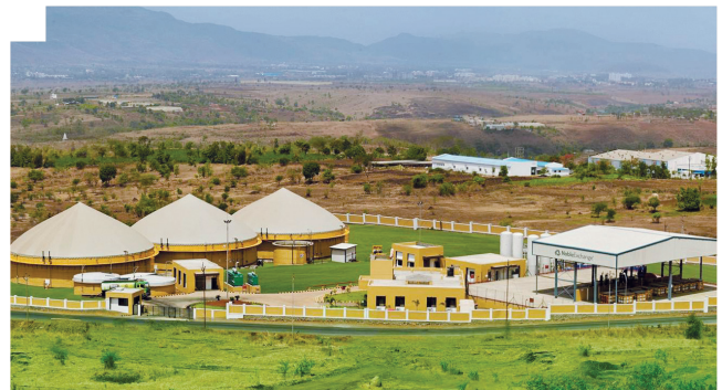
IndianOil's CBG Plant in Pune
