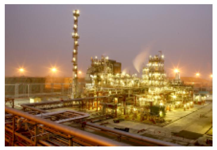
IndianOil Refineries have achieved the lowest ever MBN of 55.8 during the year, against 56.3 of previous year's. The specific energy consumption at refineries is measured in terms of MBN (MBTU/BBL/NRGF), which is the amount of energy consumed in a refinery per barrel of crude processed per unit energy factor.
