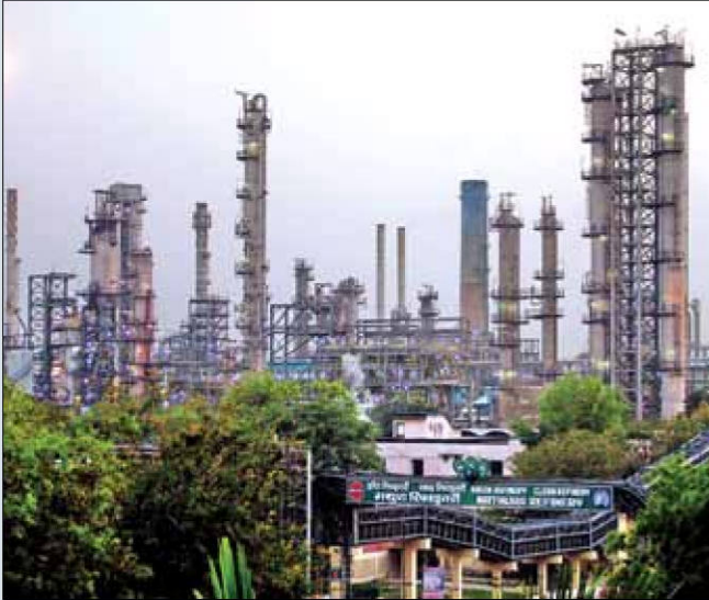
IndianOil's Mathura Refinery
