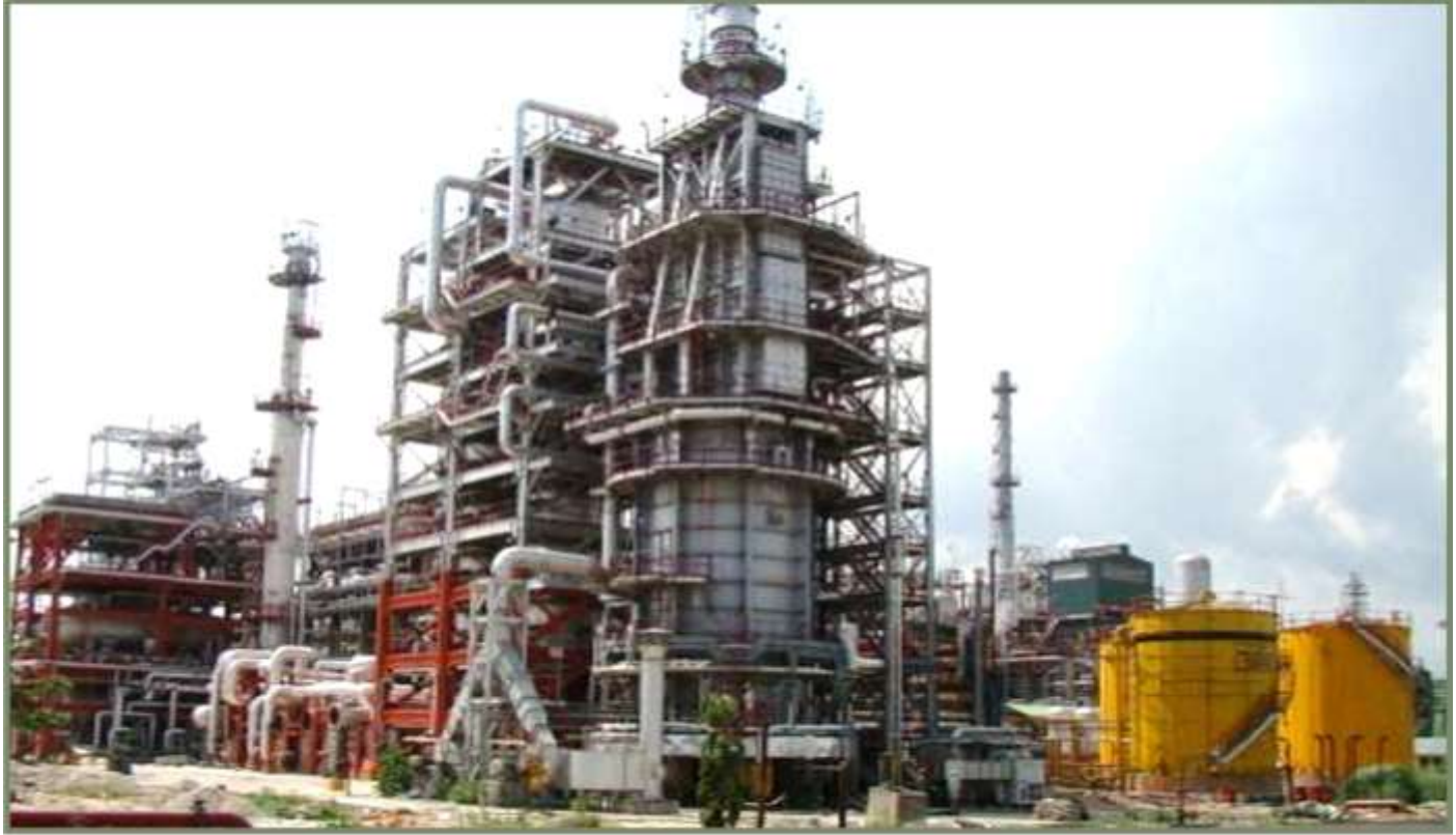
1.2 MMTPA DHT unit at IndianOil's Bongaigaon Refinery
