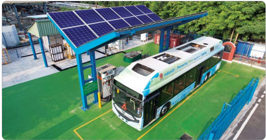
▶ Hydrogen Fuel Station at IndianOil R&D Centre in Faridabad, Haryana
