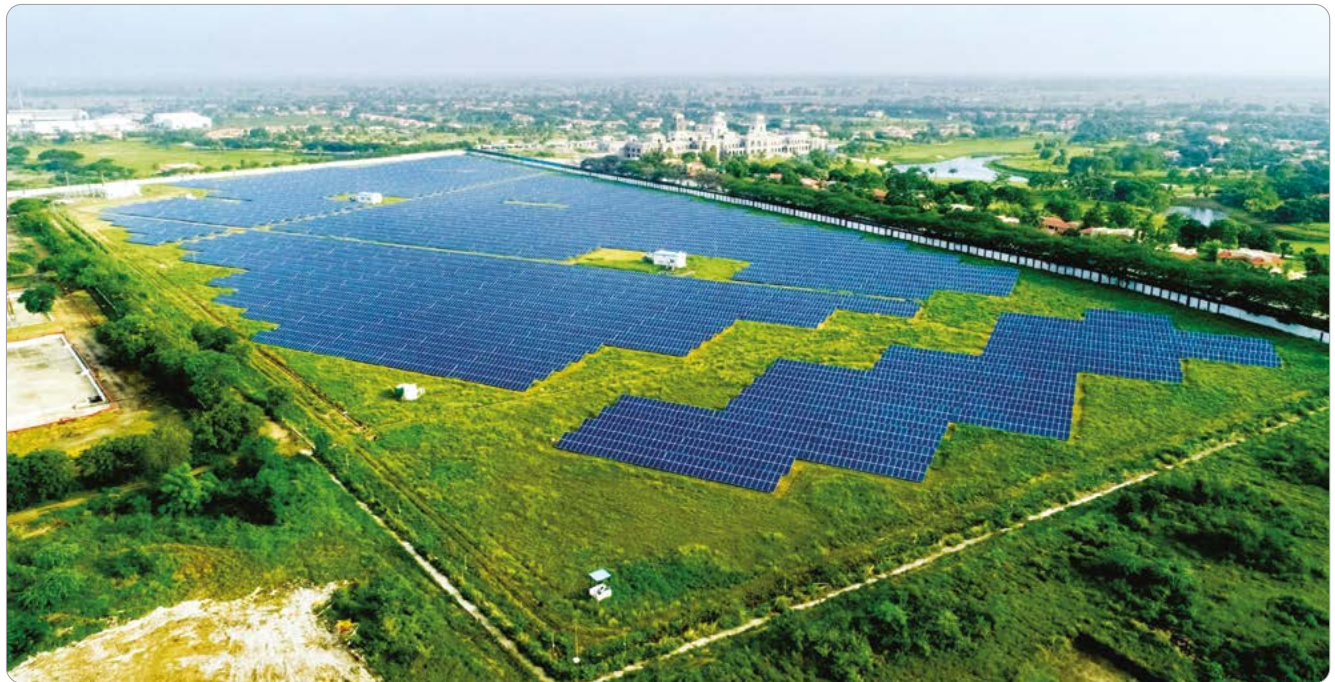
Solar power plant at Sanand LPG Bottling Plant, Gujarat
