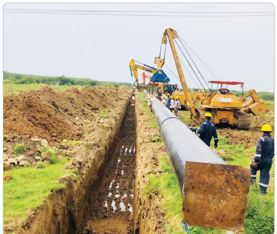
Underground Pipeline being laid in southern part of India
