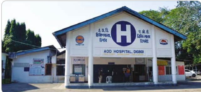
▶ AOD Hospital at Digboi, Assam
