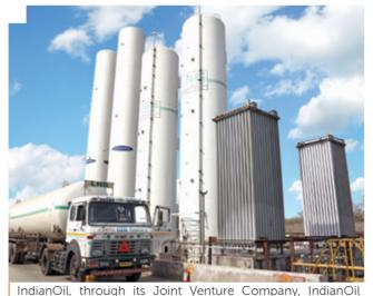
LNG Pvt. Ltd., has developed a 5-million metric tonnes per annum (MMTPA) capacity Liquefied Natural Gas (LNG) Terminal at Kamarajar Port, Ennore in Tamil Naidu
