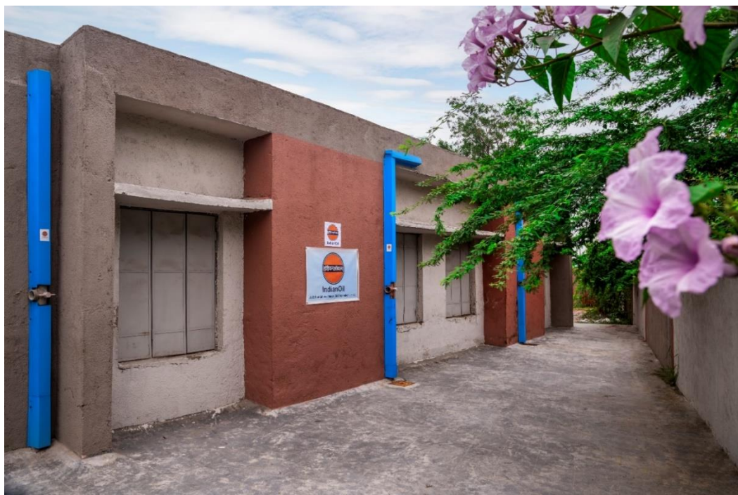
Figure 42: Rainwater Harvesting system installed in Vadodara
