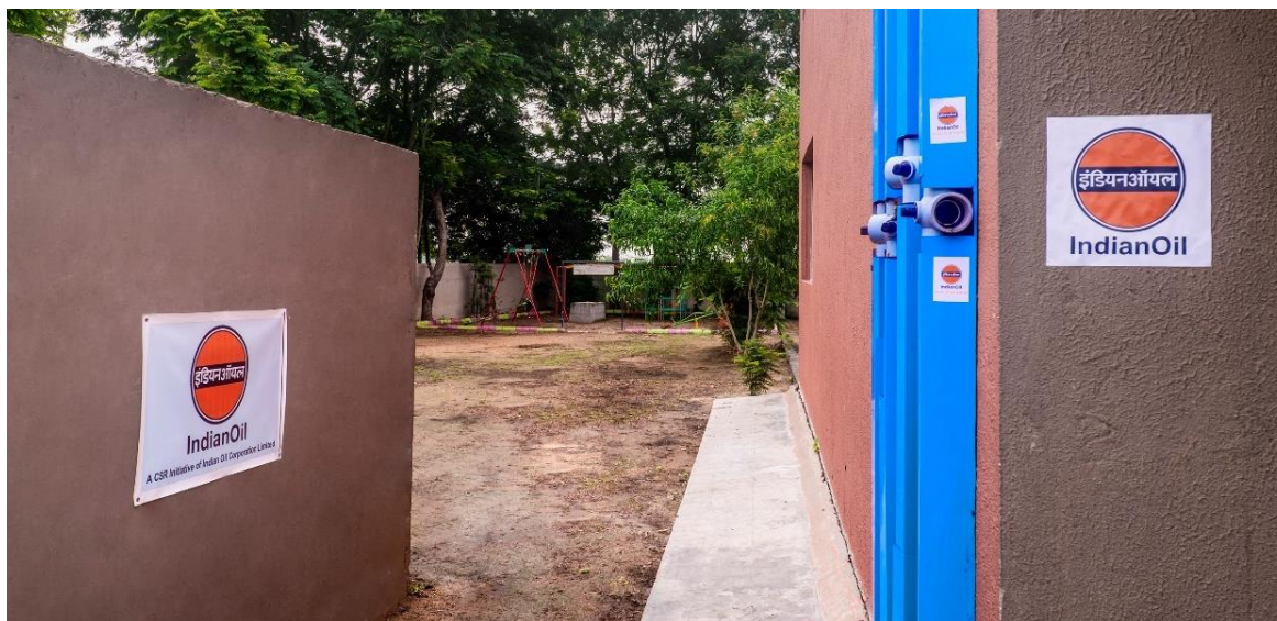
Figure 49: An exhibit of the water harvesting pipes directing the rainwater to underground
