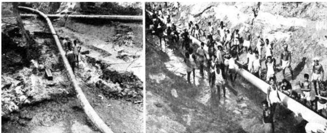
*Diversion of Damodar River submerged crossing on Haldia-Mourigram Pipeline – lowering and diverting the pipeline.*
