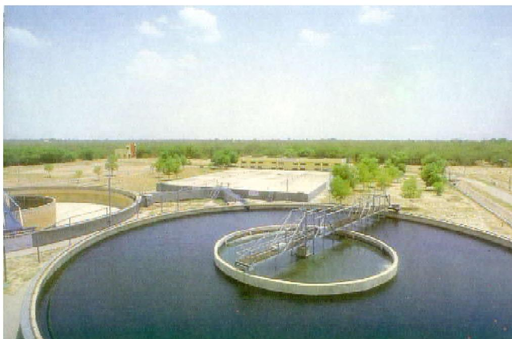
As part of environment protection elaborate effluent treatment facilities have been installed at Indianoil refineries.
