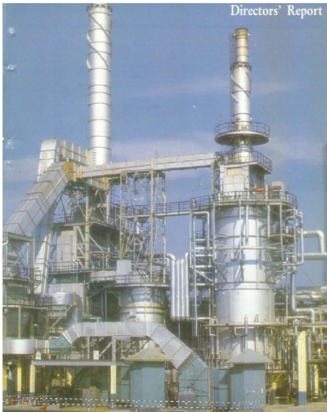
*Atmospheric vacuum unit of Barauni refinery where secondary processing facilities have also been installed to meet the increasing demand of diesel, kerosene and cooking gas.*
