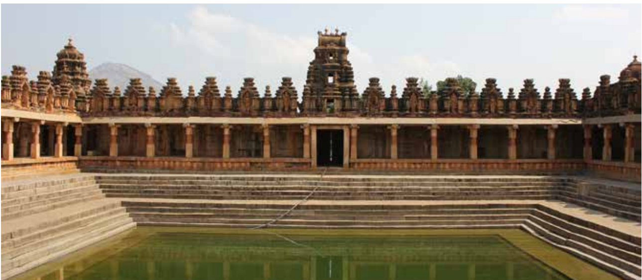
Square-stepped pond in the temple complex.
