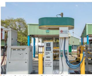
Smart Fuel Hydrogen Technology Station installed at IndianOil R&D Centre at Faridabad, Haryana
