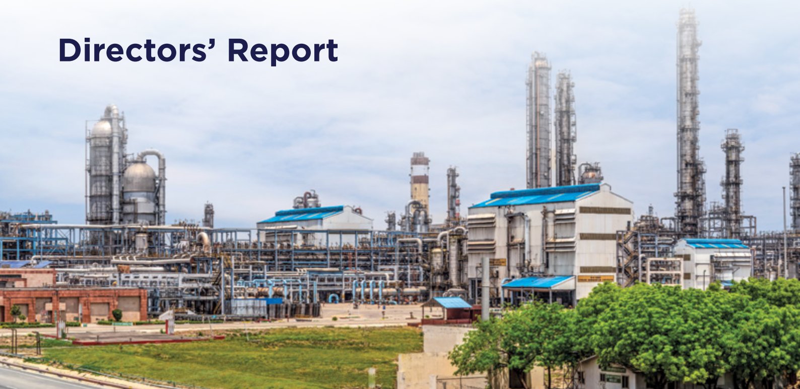
A panoramic view of IndianOil's Panipat Refinery
