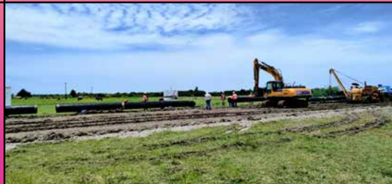
Construction work in progress for the 1,444 km-long Ennore-Thiruvallur-Bengaluru-Puducherry-Nagapattinam-Madurai-Tuticorin (ETBPNMT) NG pipeline.
