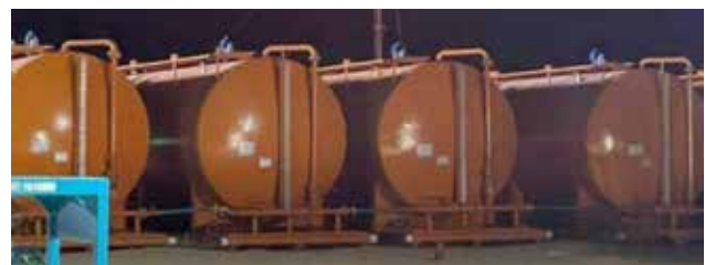
The Onshore Block 1 at Abu Dhabi.
